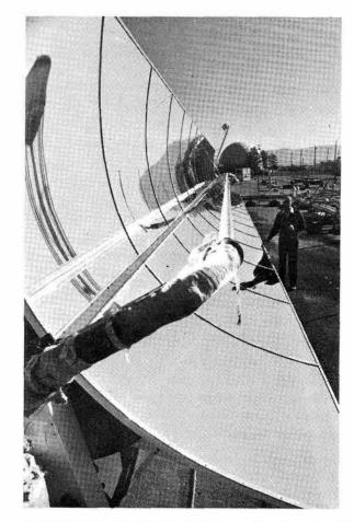
PARABOLIC TROUGH collector developed at Sandia offers highest efficiencies yet attained.
